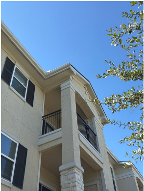
Fascia walkthrough photo 1
