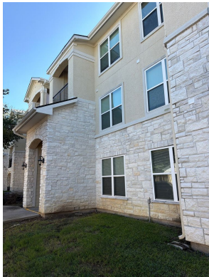
Fascia walkthrough photo 1
